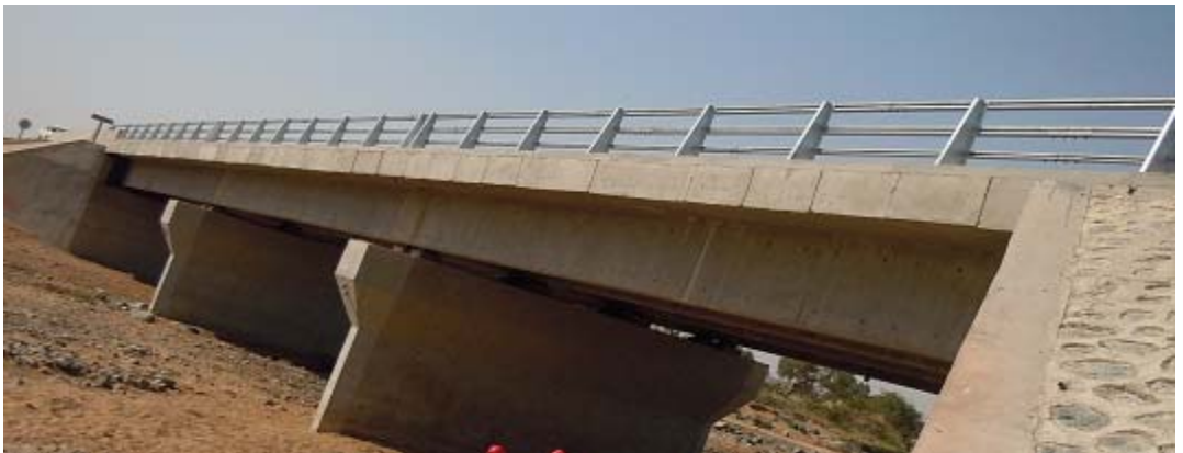
Figure 5: The reinforced concrete new bridge over the Mayo-Boula River
